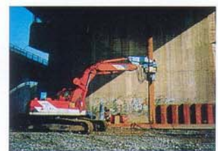
Pile is hammered and driven in place
