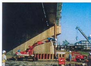
Pile is hammered and driven in place
