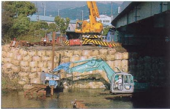
Piling in the water under a bridge
