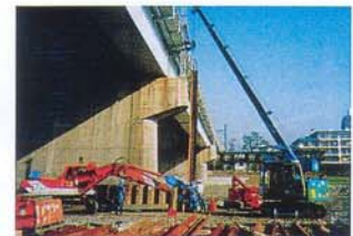
Suspended pile chucking
