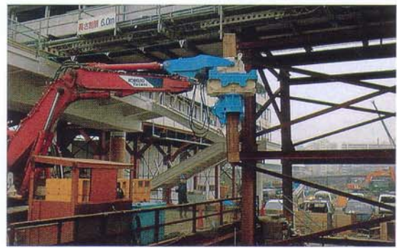
Piling in a narrow working space under a girder
