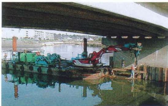
Piling in the water under a bridge
