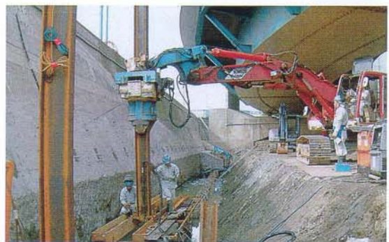
Piling in a narrow working space on an uneven ground
